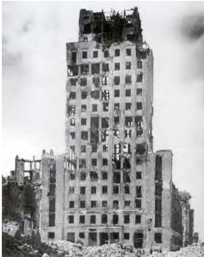
The Prudential building in Warsaw following its destruction – only the steel construction remained. Photograph taken by L.Sempolinski.
