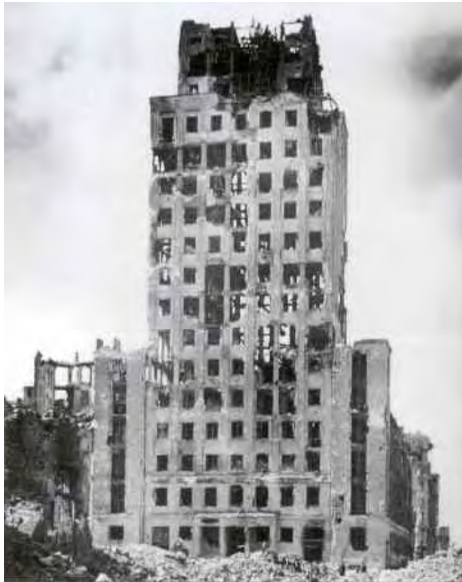
The Prudential building in Warsaw following its destruction – only the steel construction remained. Photograph taken by L.Sempolinski.
